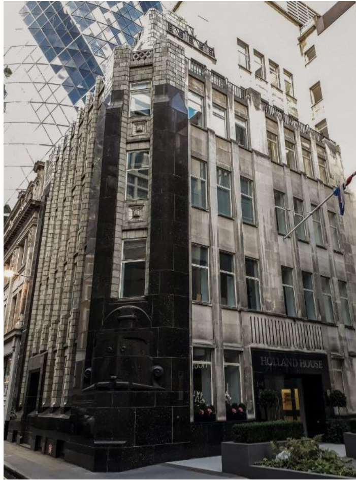
Figure 9: View of Holland House (southwest elevation) from Bury Street.
