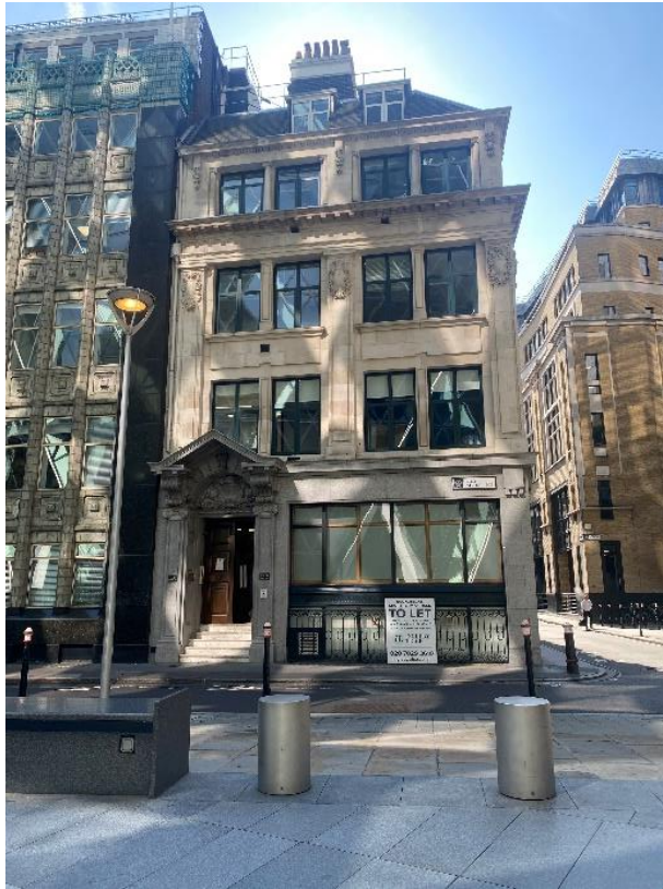
Figure 7: View of Renown House from St Mary Axe plaza.
